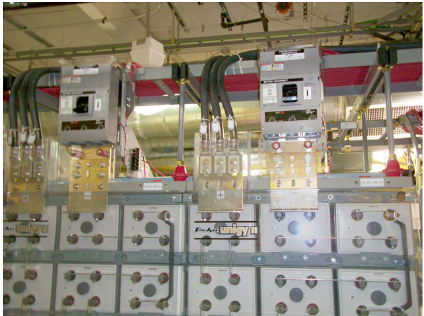
Typical 1200 Amp Top Mount Installation
