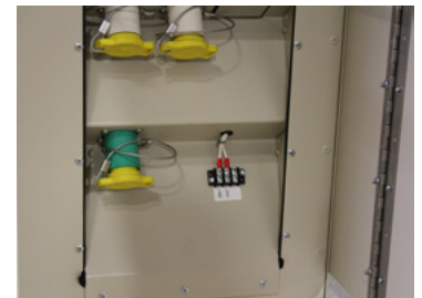
Optional Engine Start/Stop Connection
