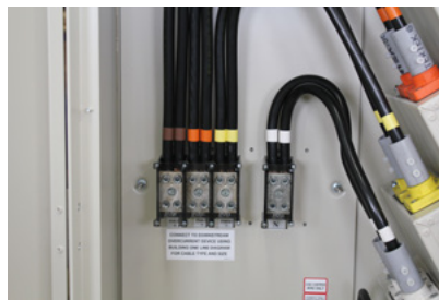
200-600A PGCB in Nema 3R Enclosure
