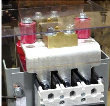
**FIGURE 6 – Disconnect with Integrated Metering Shunt**
