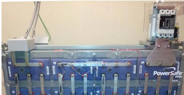
**FIGURE 3 – Disconnect Terminated on Negative Pole**
